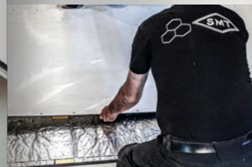
Installation of Flooring System
