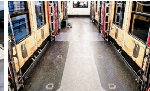
Installed Flooring System
